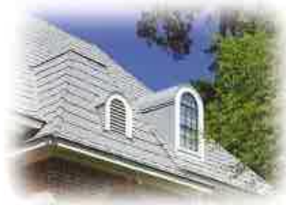
Residential Metal Roofing - Kingwood, TX
